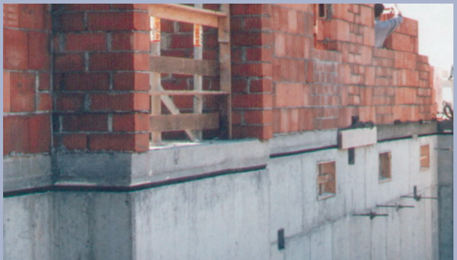
Figure 2: Stripped and finished horizontal joint
