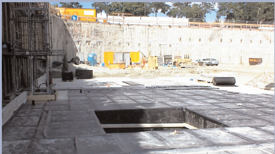
Installation of CIMAX
