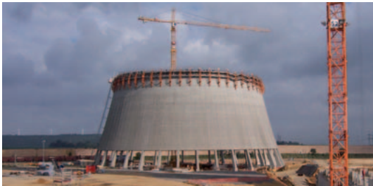
Power plant under construction
