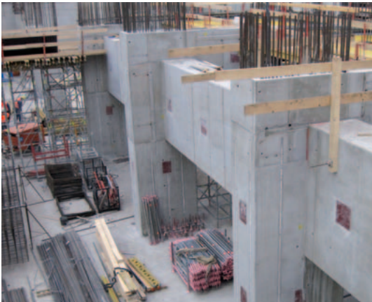
Anchor channels in elevator shaft or stairway
