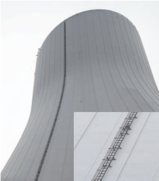
Fastening of exterior ladder
