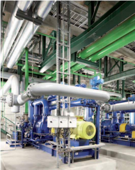
Fastening of heavy machinery
