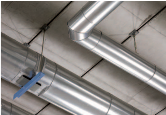
Fastening of heavy duty water pipes
