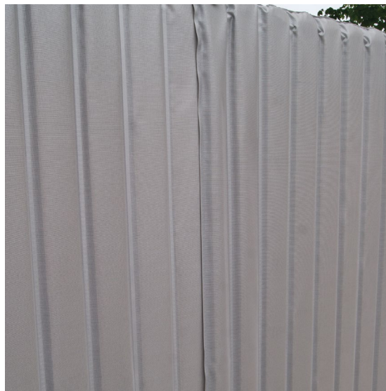
Figure 6: Edges overlap to provide a seal
