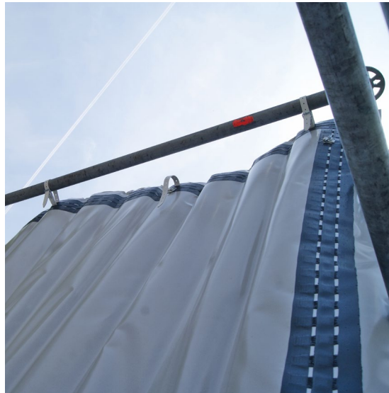
Figure 4: Fastened and aligned
