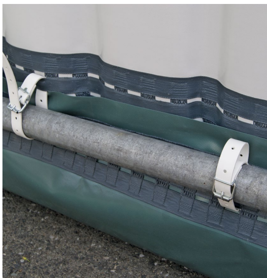
Figure 8: Fastening protective strip to scaffolding pole
