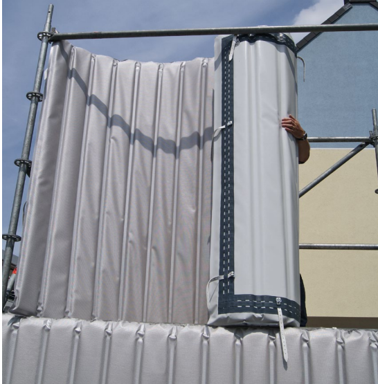
Figure 3: Unrolled in a scaffolding section
