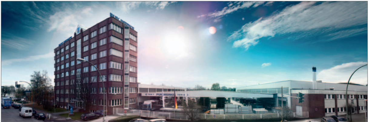
The JORDAHL headquarters and service centre are based in the same building as our affiliated company PUK
