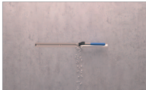
Remove anchor channel foam fill with the aid of a suitable tool
