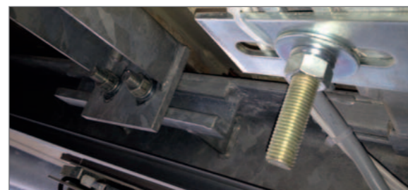
Securing lift doors in a lattice girder shaft
